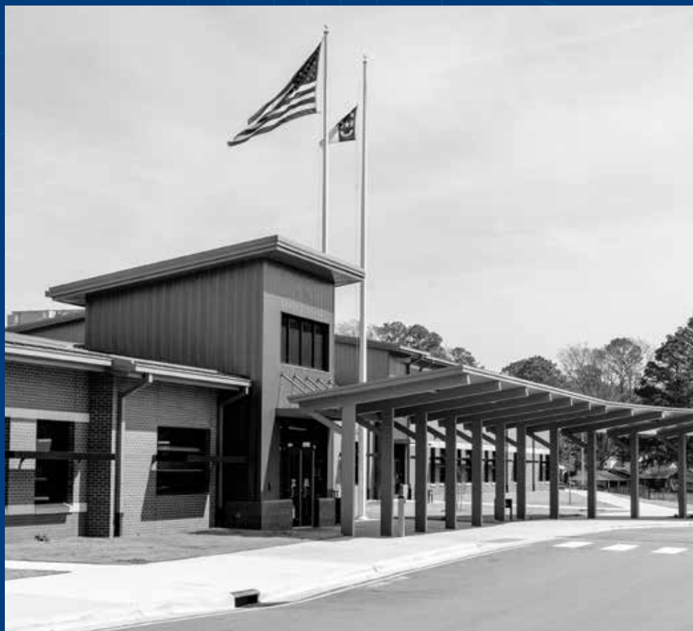
New Ahoskie Elementary School, Hertford County
